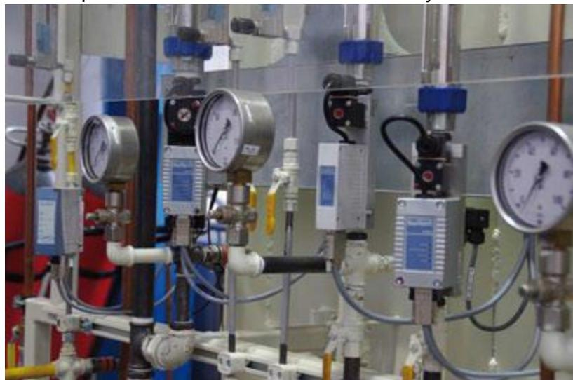
Fig. 2: Flow controller installation for control of process gases and liquids
