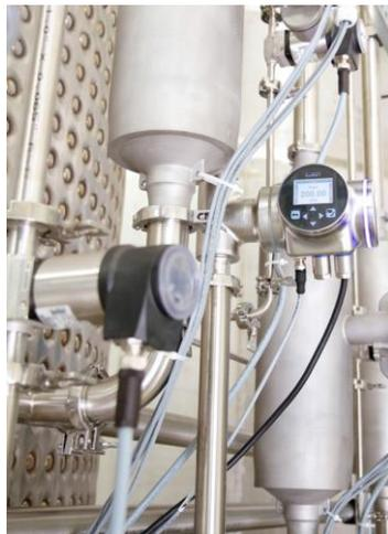
Caption 2: FLOWave enables continuous monitoring of the cleaning procedure, which makes it a valuable quality assurance tool.
